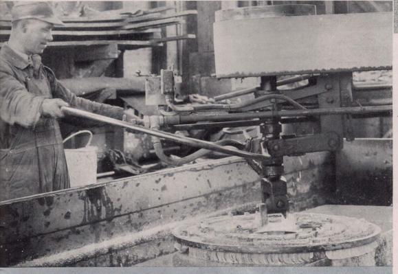
Polishing dark Select Barre Granite. Four polishing materials are necessary to produce this highly polished surface. Steel shot; coarse emery; fine emery; and last, putty powder and a felt disk.
