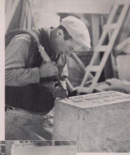
Cutting raised letters on a Select Barre Granite marker with a pneumatic tool. Great precision is necessary to do a perfect piece of work. All workers on Select Barre Granite are highly trained artisans.
