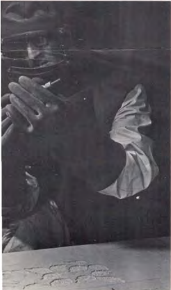
4. Preparing to shape-carve a design in Barre granite by means of sandblasting.
